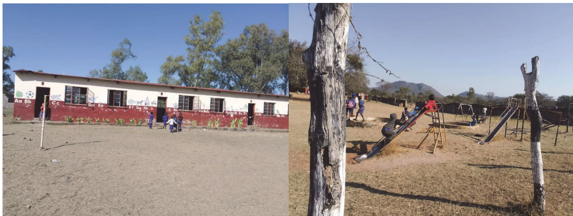
A 3-roomed classroom block and an outdoor ECD play centre with child-sized play equipment
