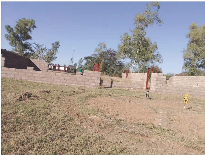
The ECD block still under construction
